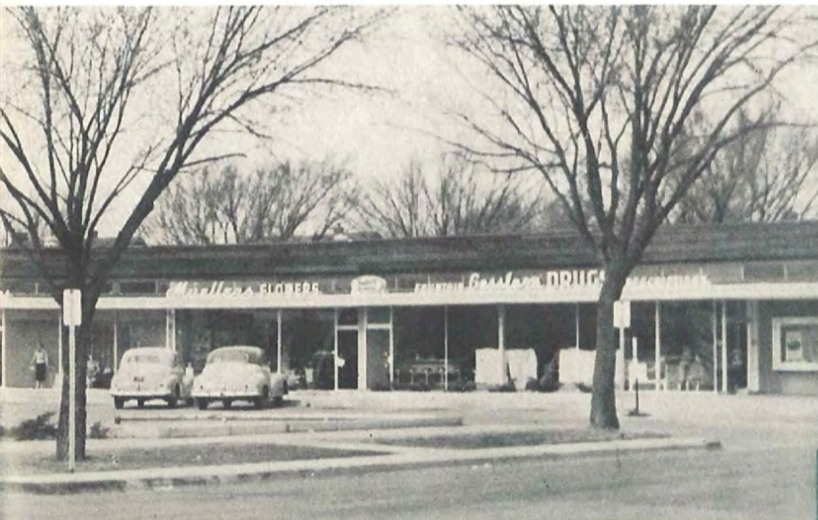
Location: Wichita, Kansas. Architects: Forsblom & Parks, Wichita.
