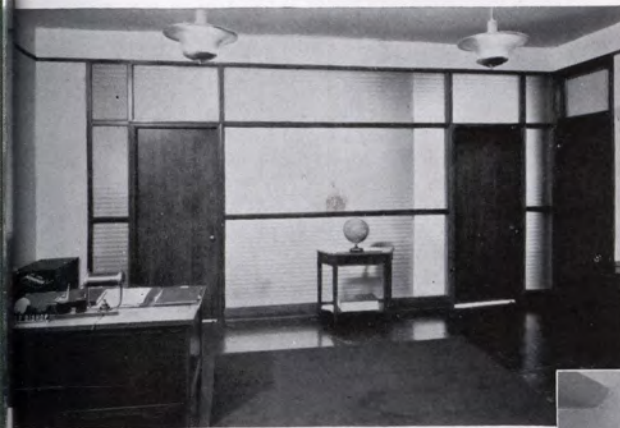
ABOVE: A bright, attractive office is screened from the reception room in the offices of the E. J. Hunt Company, Detroit. The glass is double-glazed Louvrex with Satinol finish on the outside to absorb reflection.
