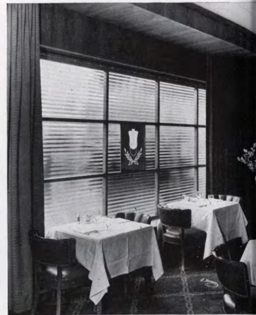
ABOVE: The same windows as shown above in the Grenadier Dining Room and Bar, seen from the dining room. Notice how ample light is provided through the large panels of Louvrex without sacrificing privacy.
